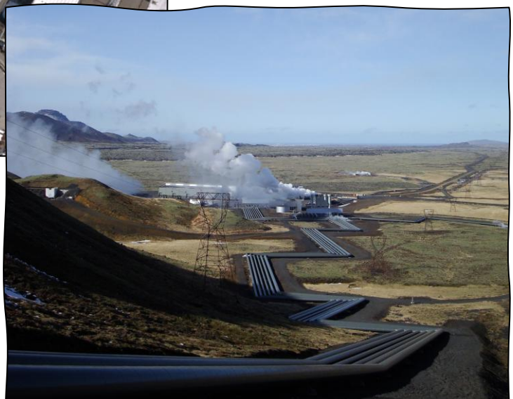
Figure 9. The Hellisheiði power plant in Iceland generates electricity and hot water using 50 boreholes that reach depths of up to 2,200 metres. (© ThinkGeoEnergy, CC BY 2.0, https://commons.wikimedia.org/w/index.php?curid=10907139 )
