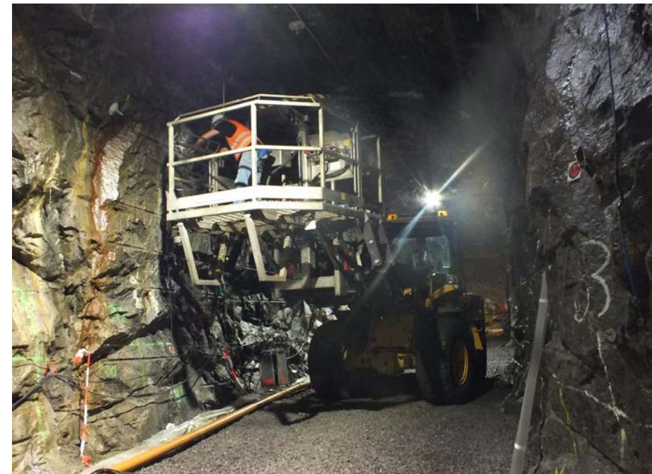
(b) Roof installation of AE sensor
