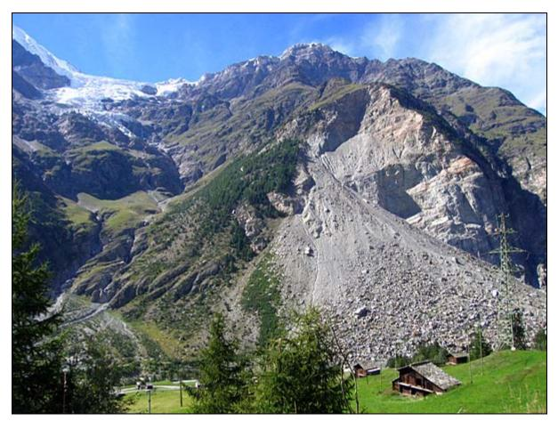
Figure 2: Detail of the scarp and deposit of the 1991 failures at Randa.
