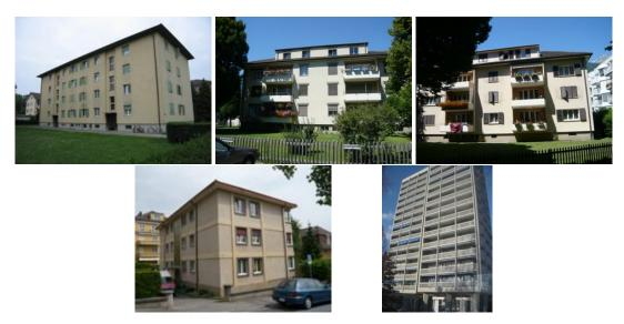
Figure 11: Picture of the URM buildings built before 1970 (#8,9,10,11,12).
