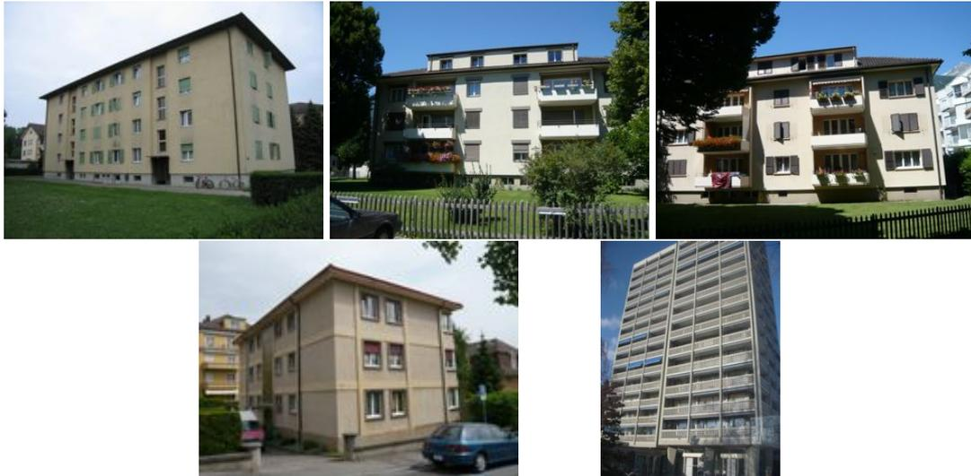
Figure 11: Picture of the URM buildings built before 1970 (#8,9,10,11,12).
