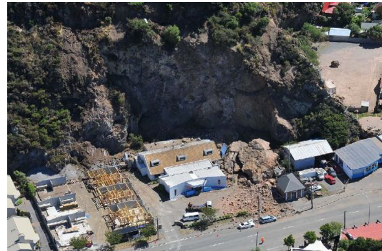
Photo 6. GTH_5708 (Rock falls RSA Building in Wakefield Ave Sumner (rock fall fatality reported at building site left).
