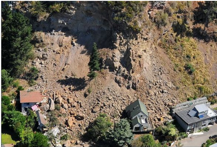
Photo 17. GTH_5787 - House destroyed by rock fall at 54 Raekura Place, Redcliffs (reported fatality site).
