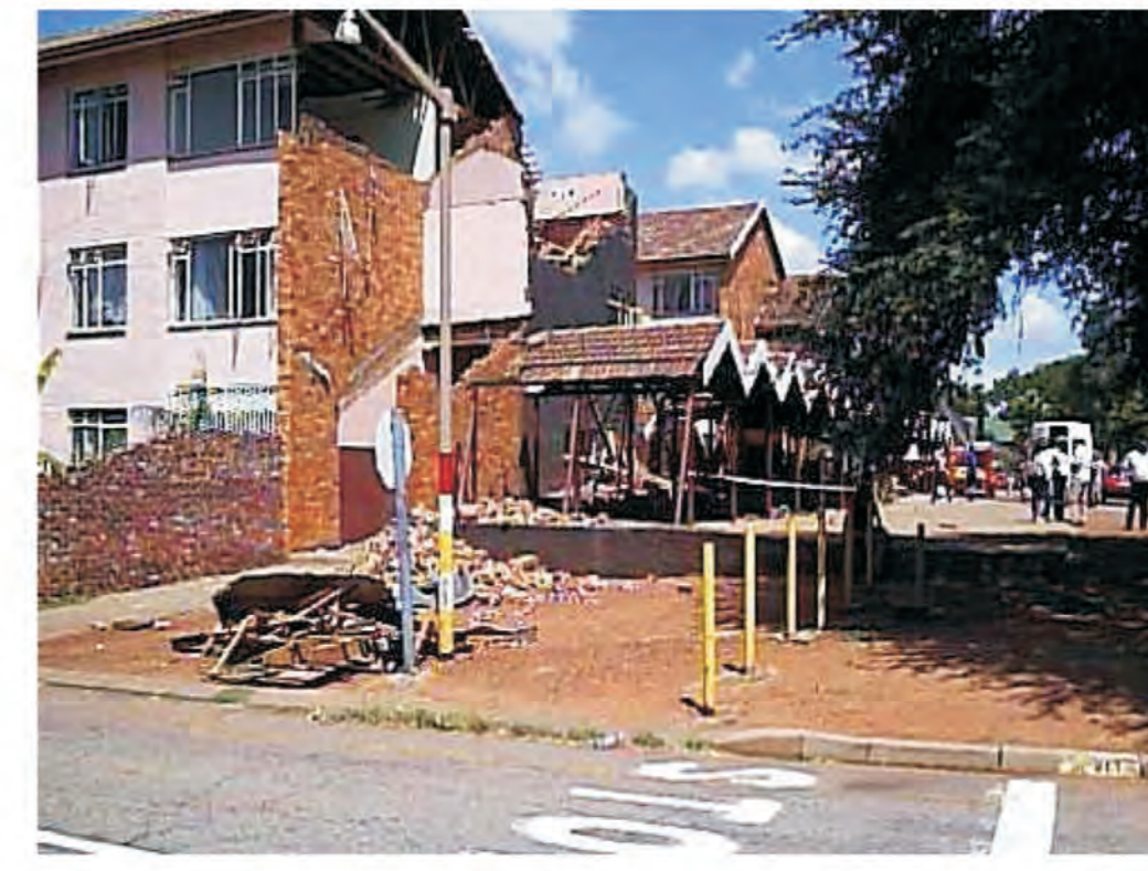
Fig. 2 Damage to a building caused by mL 5.3 rockburst from March 9, 2005 in Stilfontein, South South Africa (courtesy of dr A. Cichowicz, South African Council for Geoscience).
