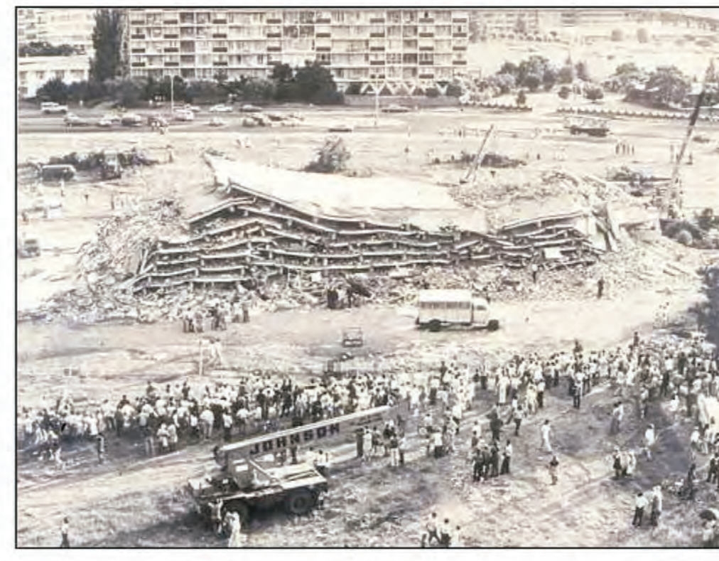
Fig. 1 Collapsed building in Welkom (South Africa) caused by mL 5.2 rockburst from December 8th 1976 (courtesy of dr A. Cichowicz, African Council for Geoscience).
